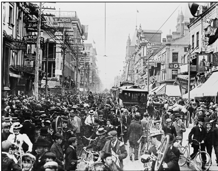
Yonge Street looking north from Adelaide Street, 1900 (Galbraith Photograph Company n.d.)
